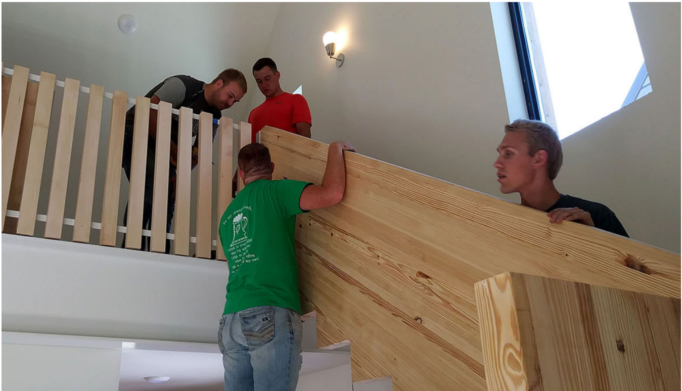
Figure 4. Student design-build stair installation at PH01:BRK. Image by author.
